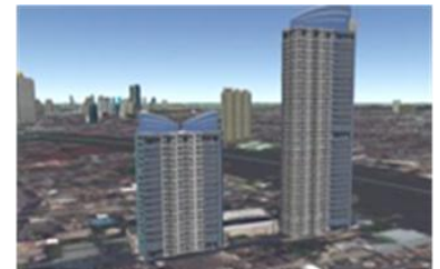
WaterMark and Chatrium Condominium Towers, Bangkok
